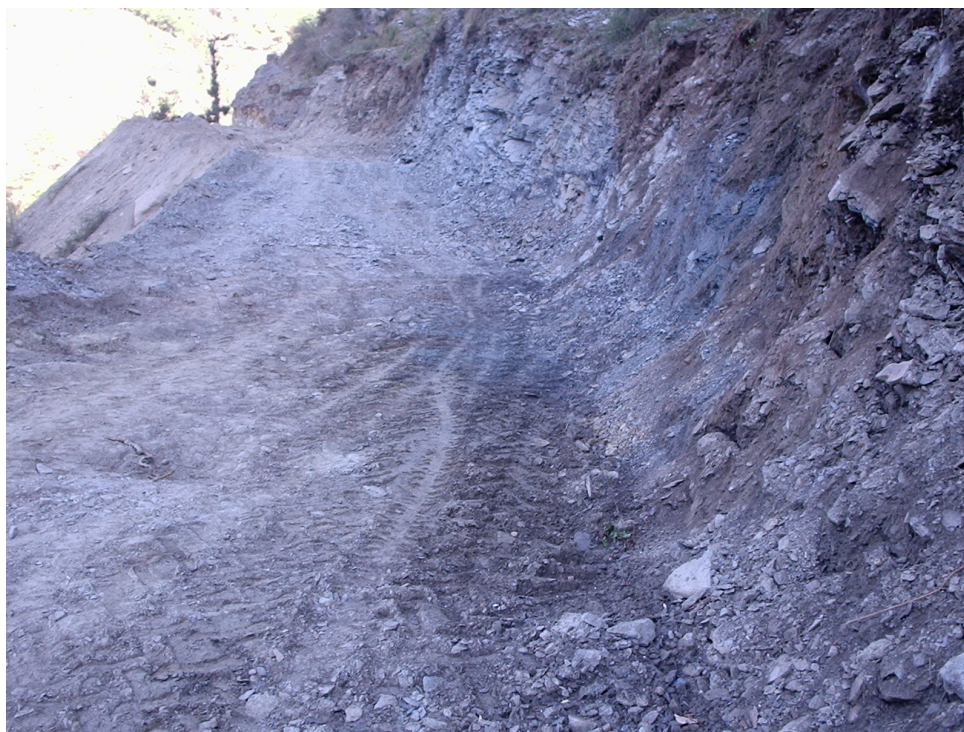
Approach road during construction stage
