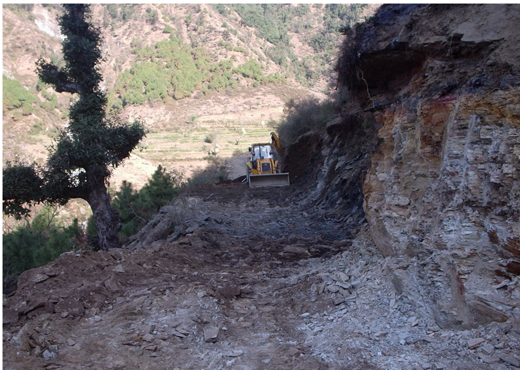
Approach road during construction stage
